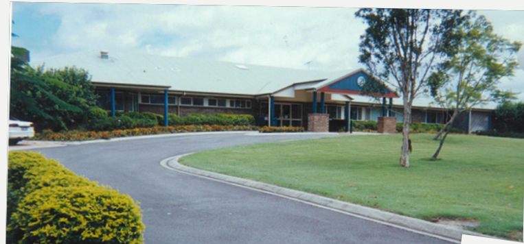
St Paul's Aged Care entrance soon after completion.
