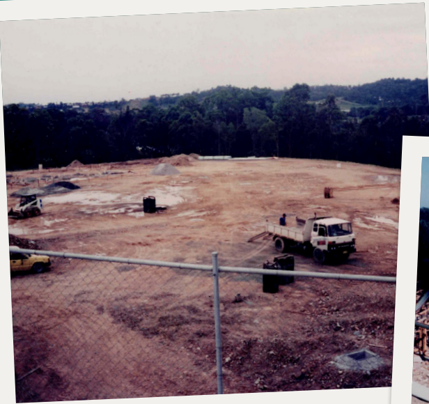
Work starts on the Tallebudgera site.
